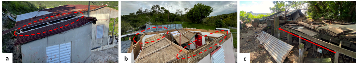
Figure 1. Damage photos showing (a) roof envelope, (b) roof-to-wall connection, and (c) sliding failure modes after Hurricane Maria (2017). Photos: Emily Alfred, Protechos.
