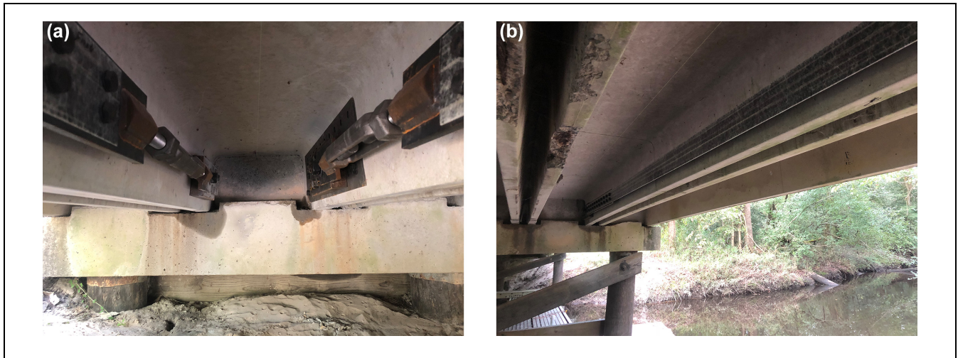
Figure 9. Overview of Bridge No. 810003 retrofit: (a) view of live-end and (b) overall view.
