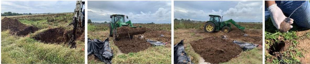
Figure 1. Construction activities and instrumentation.
