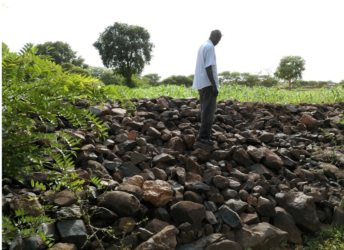
Figure 2. Level permeable dam, Commune of Kongoussi, July 2017—Photo by Colin Thor West.
