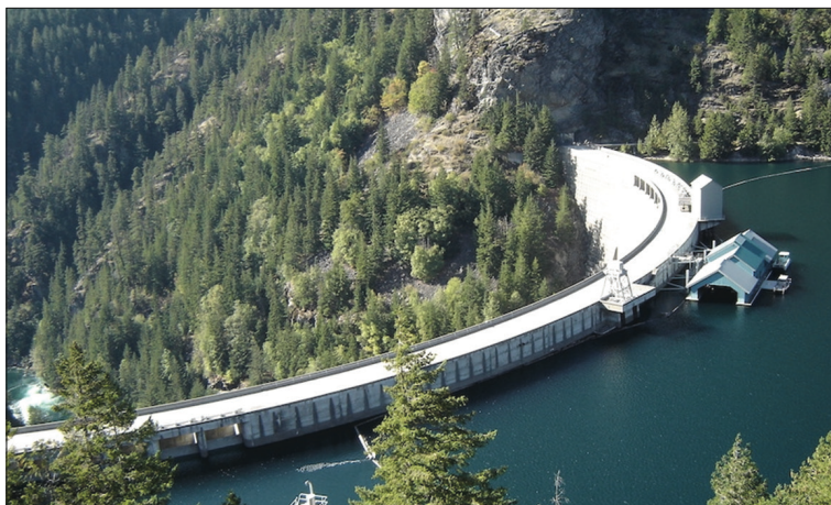
Fig. 5. One of the dams in the Skagit River Hydroelectric Project.
