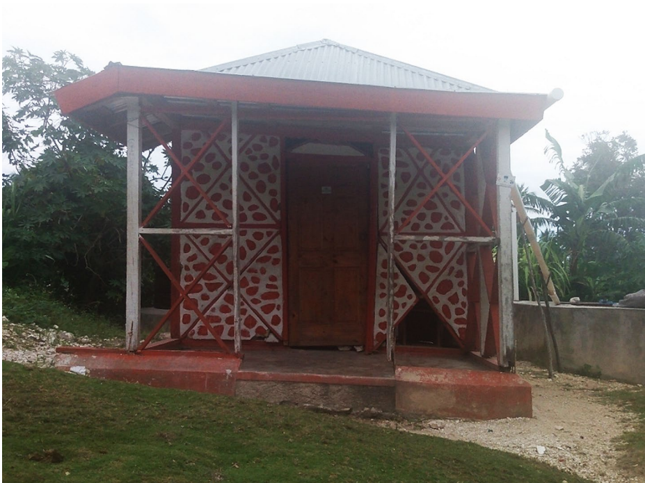
Fig. 7 Example of TCLA with minor infill loss (Fulcrum ID: a39ea13e-050c-45bb-a557-7d4e6115c9e2)
