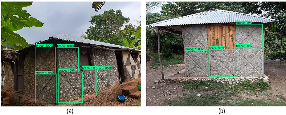
Fig. 6 Examples of bounding box detection with prediction confidence on two TCLA homes; home on the left is unfinished with braces clearly visible but braces can even be detected on the stuccoed home on the right
