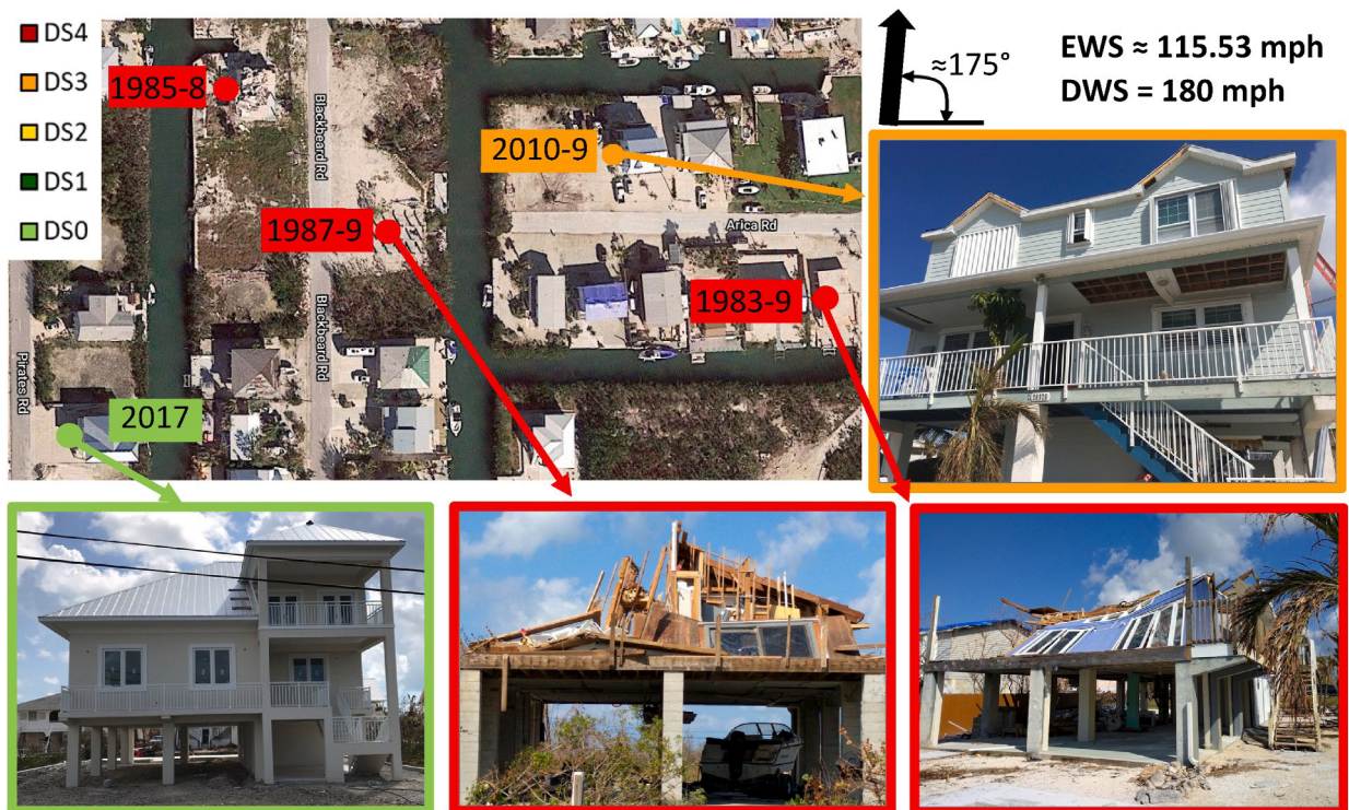
Fig. 14. Levels of wind-induced damage to construction in Little Torch Key, Florida, during Hurricane Irma with estimated wind speed (EWS) \approx 115 mph (51.4 m/s) and current design wind speed (DWS) = 180 mph (80.46 m/s) [22] (Source: NSF STEER on Fulcrum).
