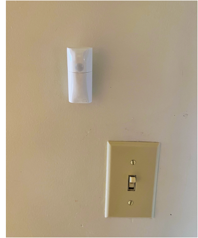
(b) A motion sensor installed on the wall of a home, by a light switch. Similar sensors were used for the ceiling.
