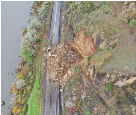
Figure 3. The landslide occurred on Oregon 138 West captured by a UAV (Source: ODOT 2021)
