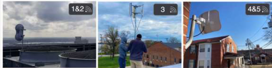
Figure 1. Five different stages in setting up a community mesh network in the urban context: (1) Point-of-Origin is created through broadcasting back-bone internet connection from Internet Exchange from high viewpoint Primary Sectors, (2) point-to-multipoint backhaul units are setup, (3) community-based geographic high points (such as school buildings) are used as Relay Sectors that receive signal from a Primary Sector and relay to nearby households, (4) household connections are setup with onsite receiver, cabling, and router, (5) (optionally) community WiFi hotspots are set up in the immediate vicinity.
