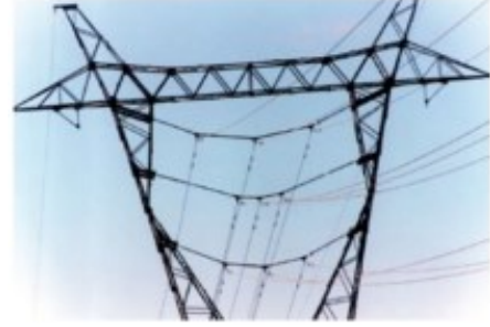
Fig. 3. Structure of the 230 kV unconventional HSIL experimental line [9].
