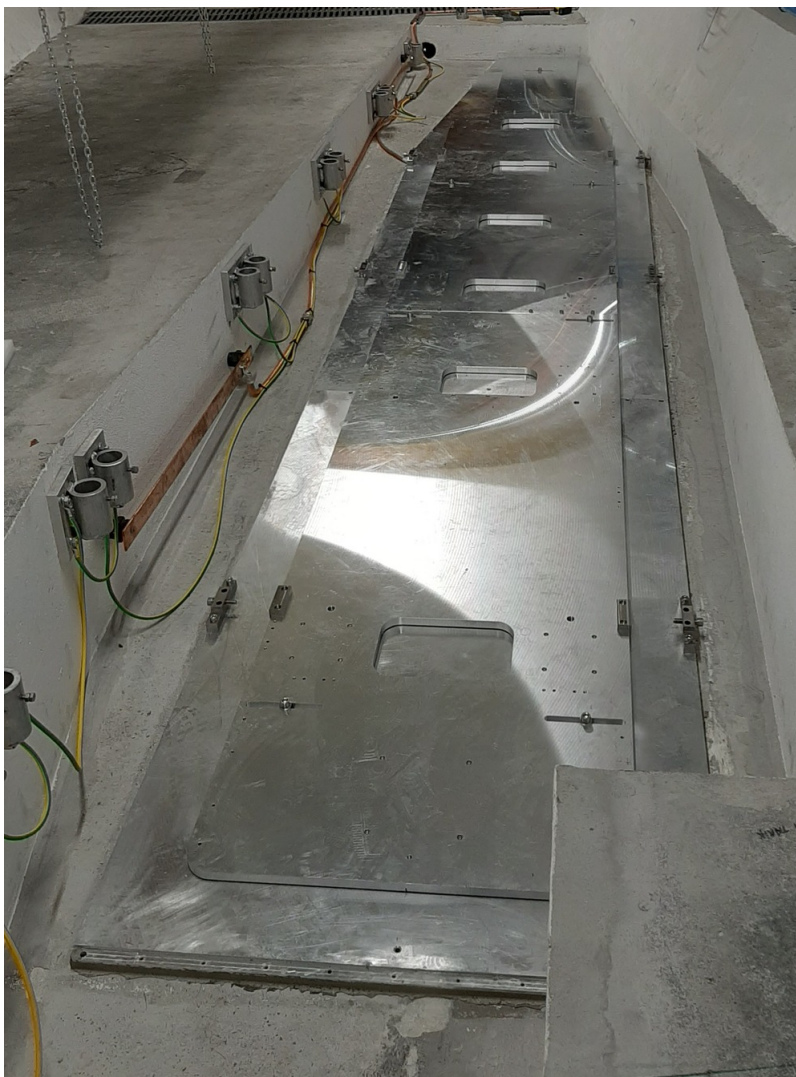
Figure 58. A picture of the upper and lower baseplates installed in the FASER trench, before the detector was installed.
