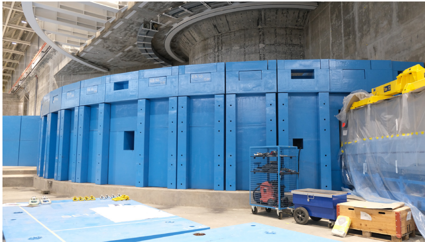
Fig. 5. The ESS bunker wall.
