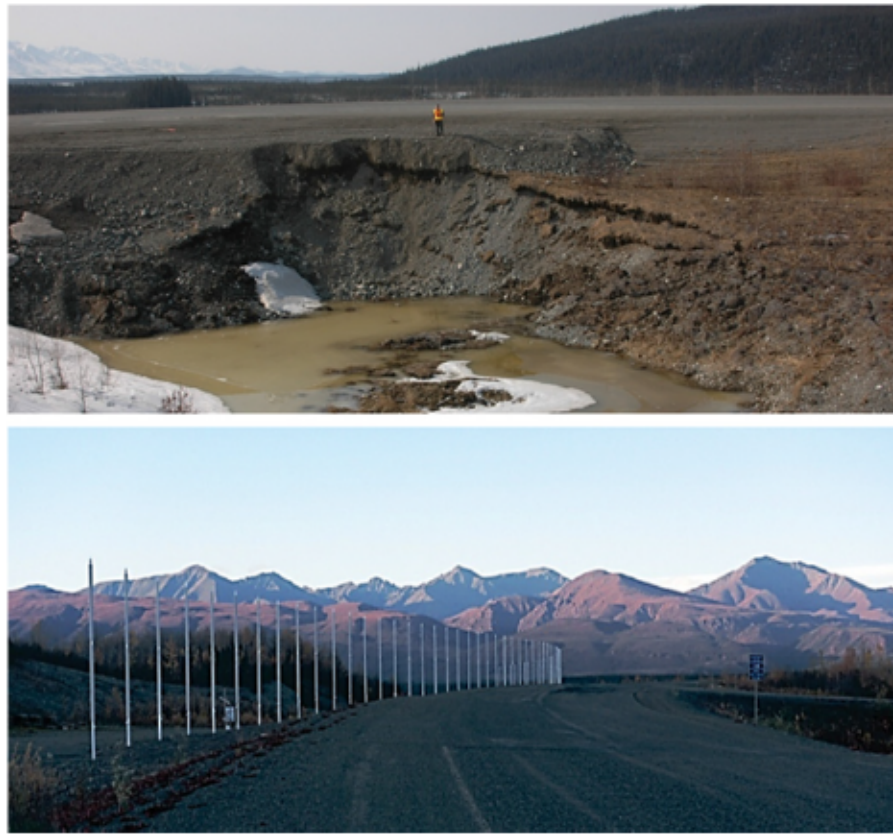
Fig. 7. Adaptive engineering to protect the Alaska–Canada Highway in a warming climate. A section that was especially prone to permafrost thawing and collapse (top; photo credit: Daniel Fortier), was rebuilt and fitted with thermosyphons to maintain the frozen state of the permafrost (bottom; photo credit: Fabrice Calmels).
