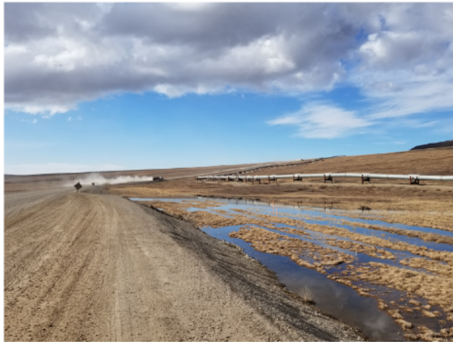
Fig. 3. Road dust and ponding at the edge of the Dalton Highway, near Toolik Lake, Alaska. Photo credit: Christopher Arp.
