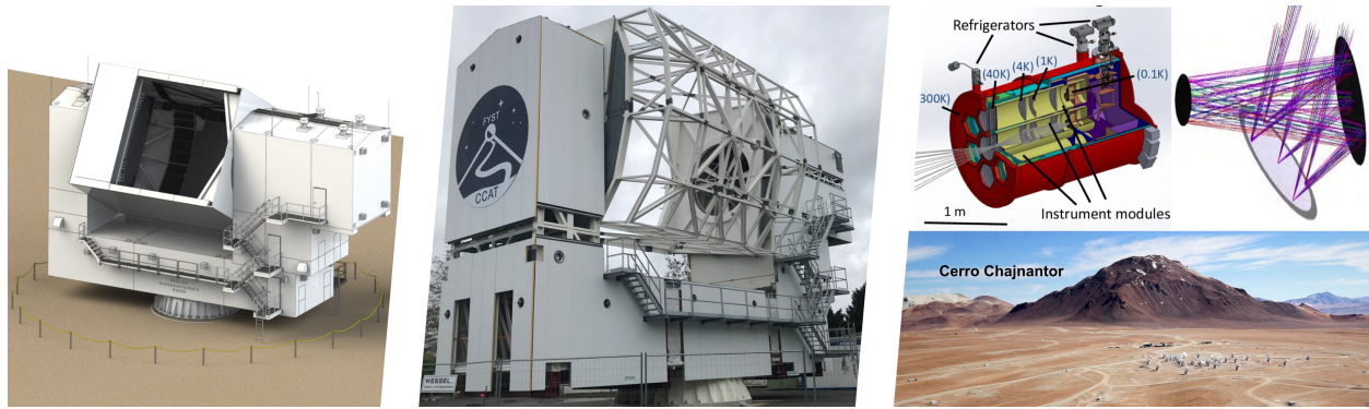
Fig 1 CCAT/FYST computer render (left), and during assembly (center). Prime-Cam and telescope optical path (top-right). Observatory site at the top of Cerro Chajnantor (bottom-right), with ALMA in the plateau below.
