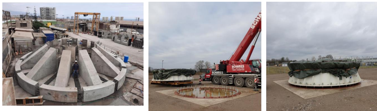
Figure 16. (left) Concrete support cone elements precast in Chile. There are 13 elements totaling 324 tons in weight. (center) Support pad prepared in Wessel, Germany, with a support ring in the background. This is the foundation for a trial assembly of the full telescope in Germany. (right) Support ring bolted onto the pad. The azimuth bearing is on the top of this ring.
