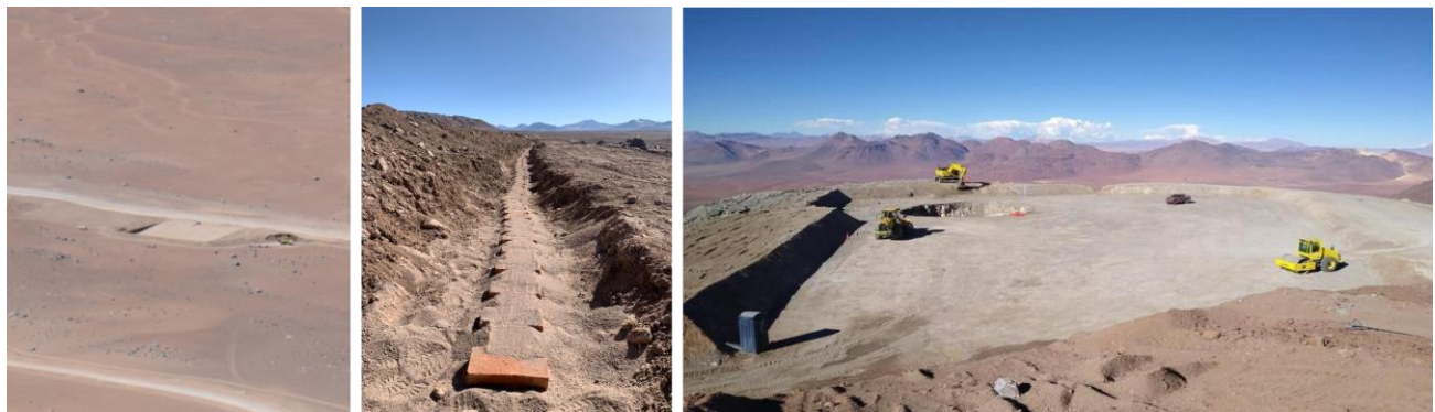
Figure 14. (left) Service area view from Cerro Chajnantor. (center) Trenching (and protective bricks) for power/data cables. (right) FYST site is leveled and the telescope foundation pour has begun.
