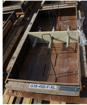
(a) mold for PG38-450-F-XL: provision of joint, hooks for lifting, dowel supports for alignment
