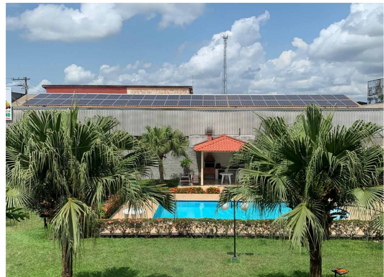
FIG 2 Due to the high prices for energy in Altamira, the city that was the host community for Belo Monte, households and businesses have started installing solar panels. A home with three bedrooms and two baths energy bills used to run up to 1,500 reais per month, after installing solar panels their bills declined to around 100 reais. A growing number of households are installing them, and the government and energy sector instead of providing incentives, will begin charging a 60% penalty to new installers in 2023 in order to discourage this sensible development.
