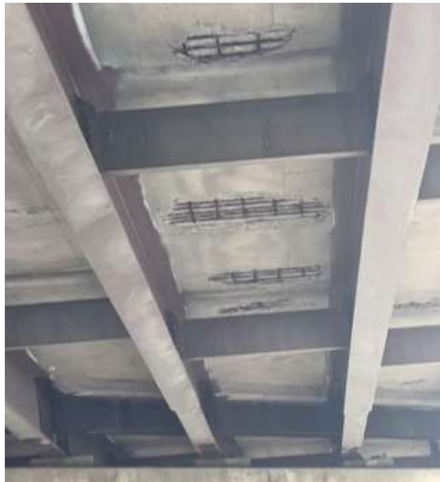
Figure 2 Highway overpass bridge with multiple delaminations of concrete on underside of the deck
