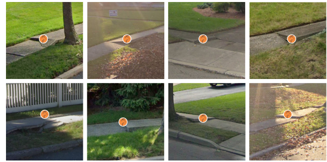
Figure 12: Project Sidewalk Oradell surface problems labels showing height differences on sidewalks and uplifts caused by tree roots.
