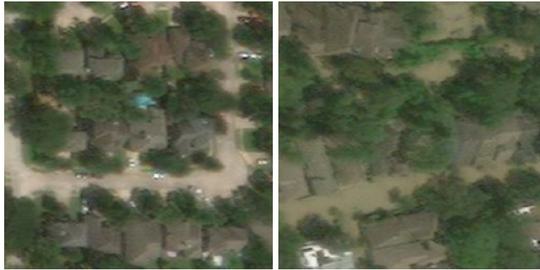
(c) ‘ Undamaged Building ’ using post-event imagery (d) ‘ Flooded/Damaged ’ using post-event imagery
