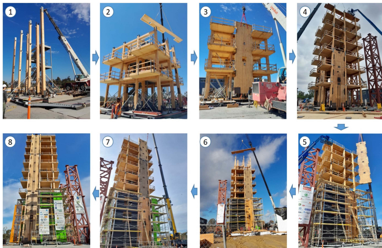
Fig. 8. Structural construction sequence of the test building. (Images by authors.)
