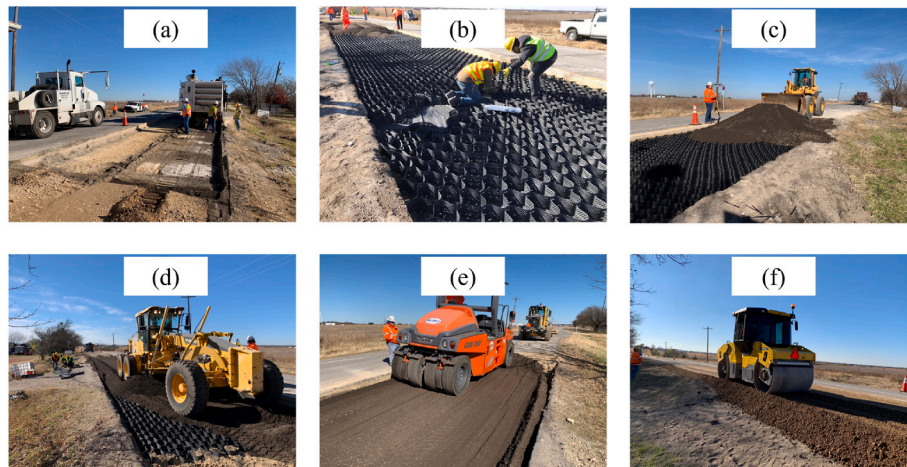
Fig. 6. Field installation sequence of geocell-reinforced reclaimed asphalt pavement base layer on FM 1807 road: a) excavation of existing road section with milling equipment; b) installation of geocell panels; c) use of excavator for dumping the RAP material into the geocells; d) use of motor grader for spreading the RAP material; e) use of pneumatic roller for the compaction of the reinforced base layer; f) use of vibratory drum roller for the temporary surface layer.
