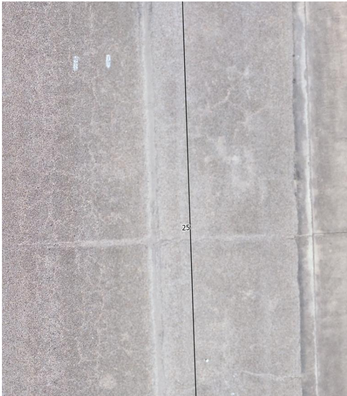
Figure 8. Early-stage alligator cracks present along Line 25
