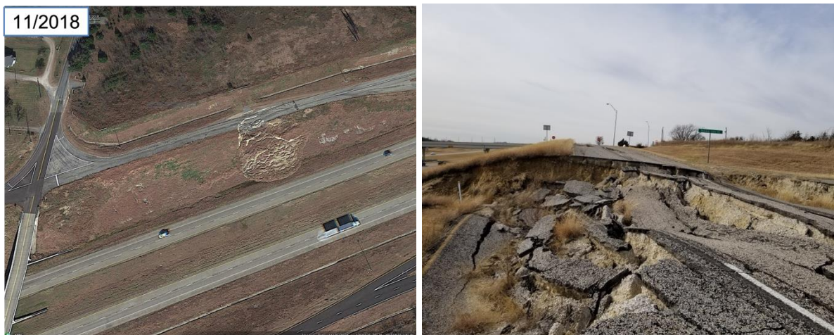
Figure 3. Propagation of severe cracks at Denison in November 2018
