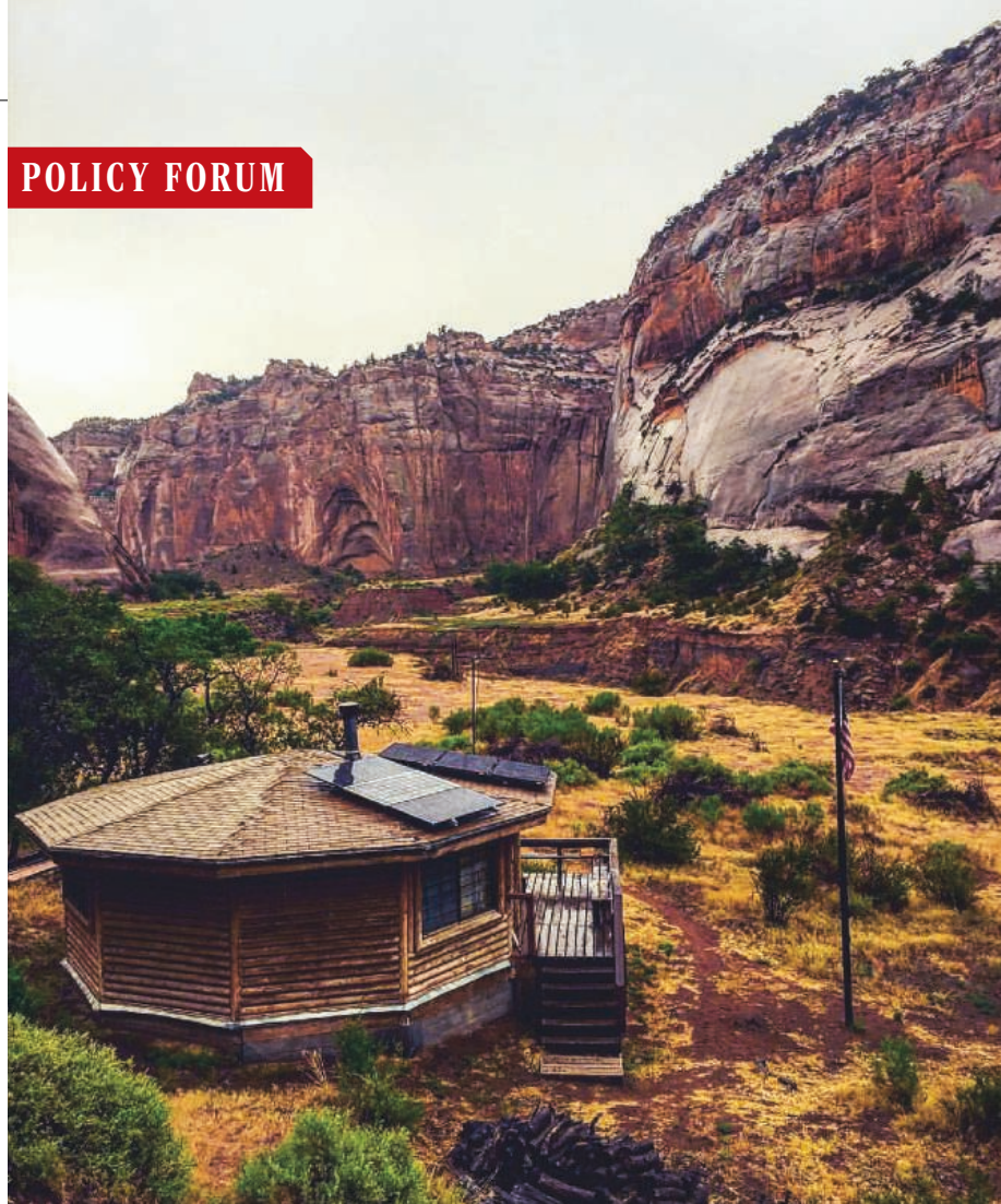
A Navajo hogan at Baby Rocks, Arizona has rooftop photovoltaic solar panels.
