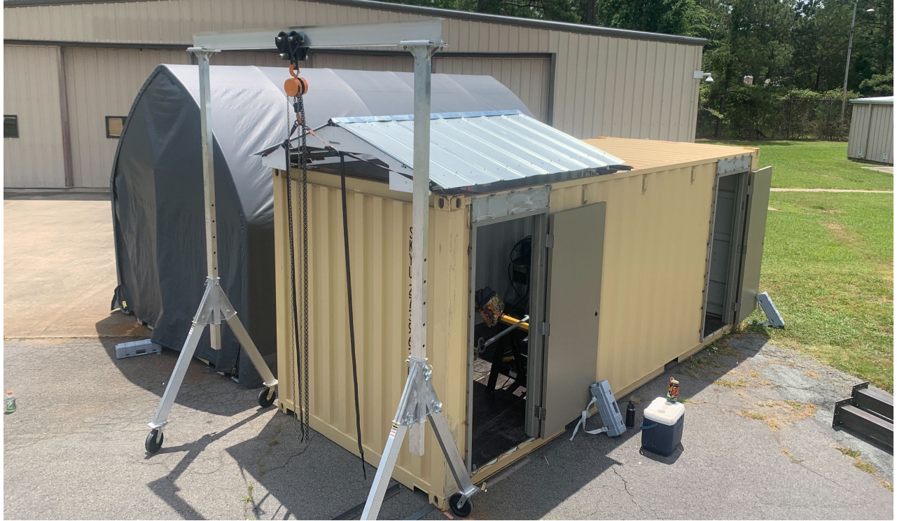
Figure 3. The nearly-complete ArgusSpec enclosure, before surface protective coatings were applied. Behind the ArgusSpec container, the Argus Pathfinder is under construction. They are built in portable shipping containers so that once construction and testing is completed on both systems they can be moved to a dark-sky site at PARI.
