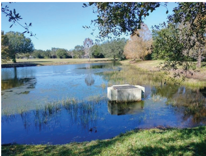
Figure 1. The concrete structure shown is an overflow structure designed to keep water below a certain level by diverting excess water to other nearby water bodies to prevent flooding. The presence of this structure indicates the water body is a stormwater pond. Credits: Michelle Atkinson, 2021, UF/IFAS
