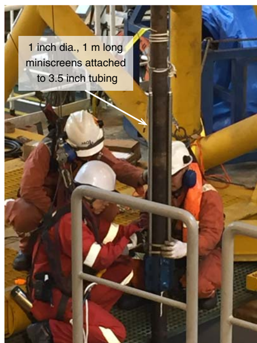
Figure F16. Miniscreens used to terminate hydraulic line at the lowermost pressure port.
