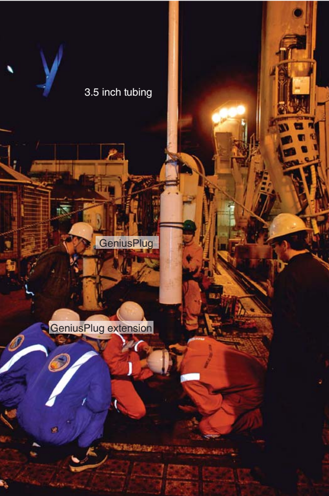
Figure F5. GeniusPlug (white paint) and tubing joints on rig floor before deployment during Expedition 332.
