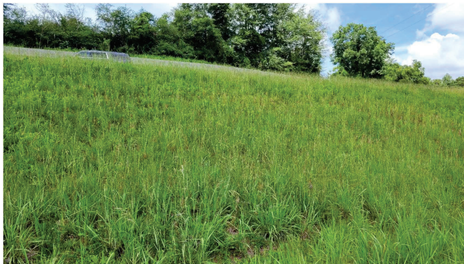
Fig. 5. Vetiver grass used to stabilize a moving highway slope in Mississippi. (Image by Avipriyo Chakraborty.)
