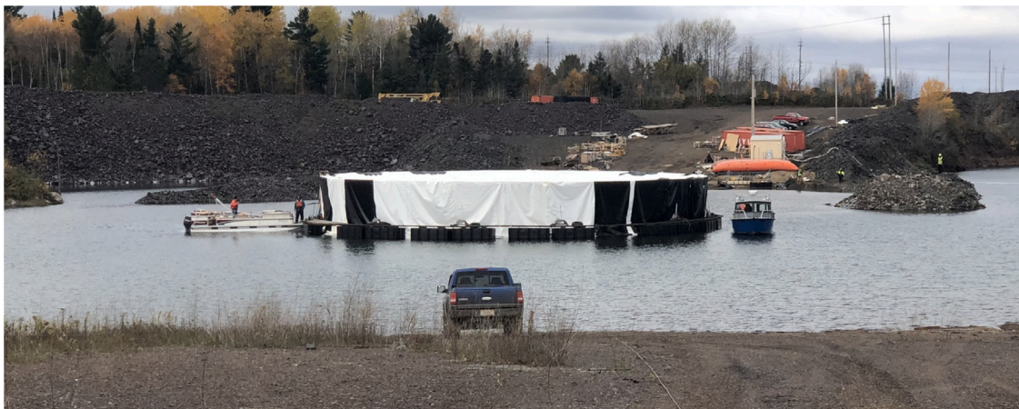
Fig. 13. The exterior of the detector after completion. The liner can be seen supporting the detector and the floating dock forms a perimeter around the detector. Two boats tow and steer the detector during deployment. The scale of the detector is visible.
