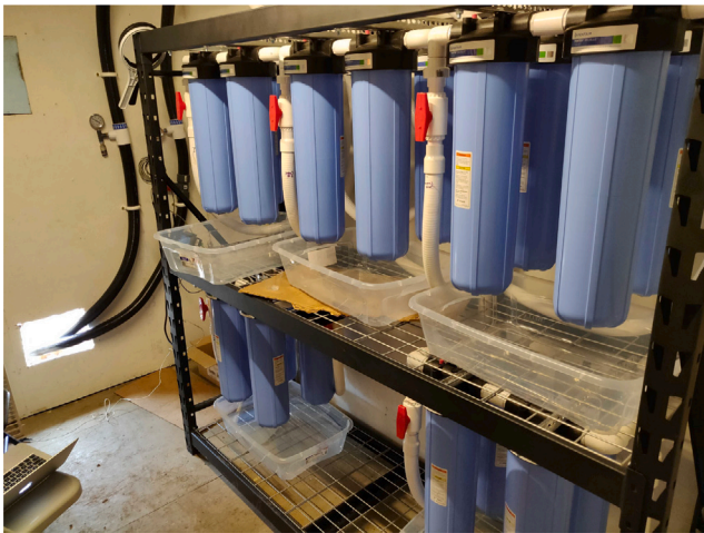
Fig. 7. The interior of the water hut showing the filtration plant.
