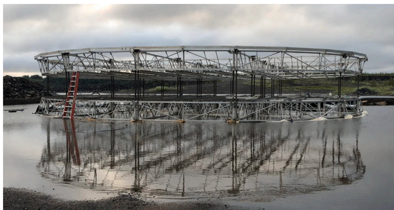
Fig. 5. Completed frame. The pillars supporting the top cap are clearly visible.
