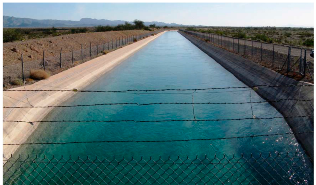
Figure 2. Canal in the Mojave Desert of California showing wildlife-proof protective fencing along the edges. Photo taken from a road across the canal.
