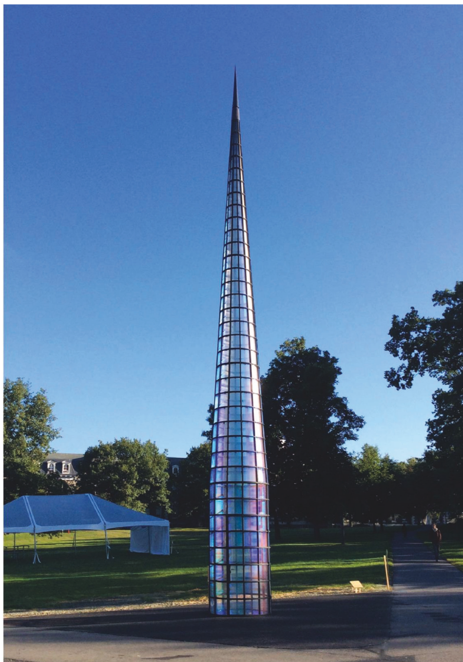
Figure 1. A Needle Woman: Galaxy Was a Memory, Earth is a Souvenir (Kimsooja). Cornell Arts Quad. Steel installation (1.3 m diameter at base, \approx 14 m height), window panels coated with iridescent self-assembled lamellar block copolymer film whose lamellar sheets were oriented vertically along the tower long axis. Today, this structure is part of the permanent museum collection at Yorkshire Sculpture Park in Wakefield, UK.
