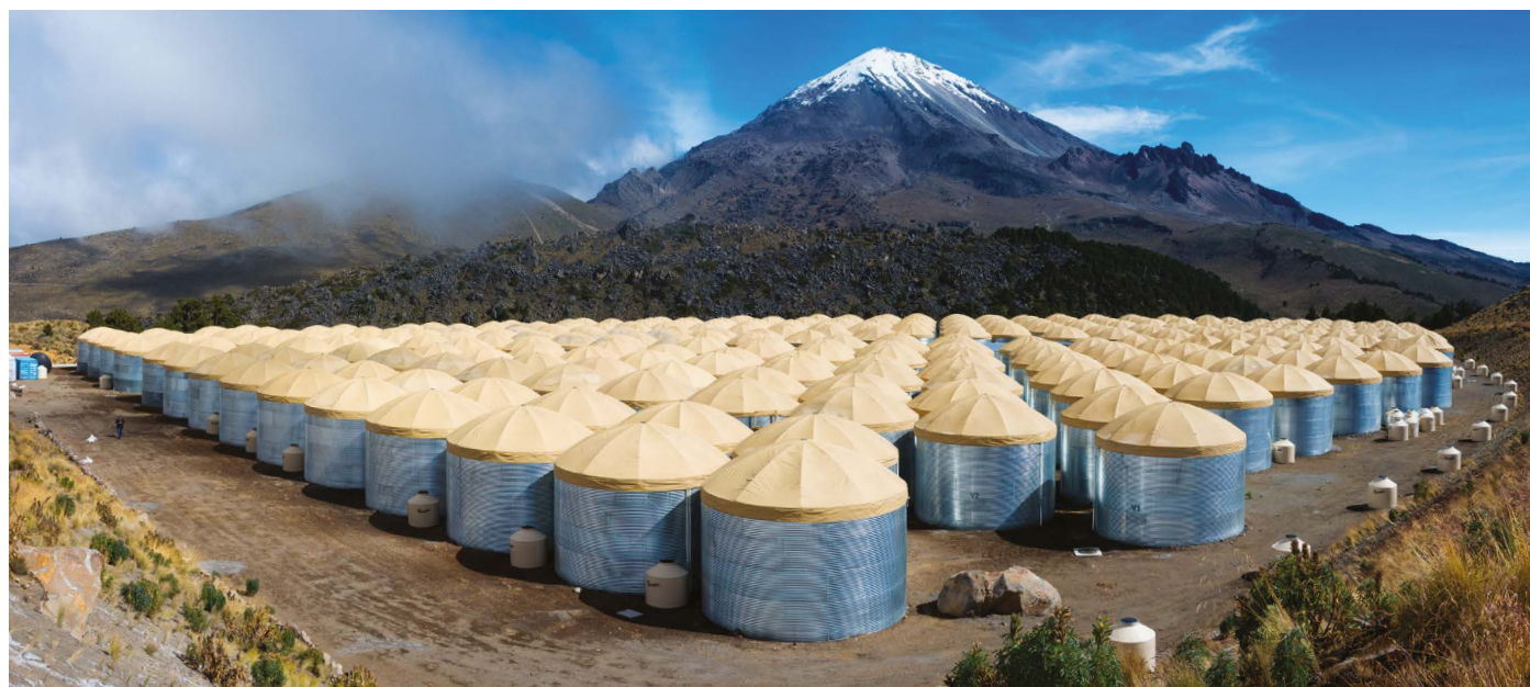
Figure 1 | Detecting \gamma -rays from microquasars. The High-Altitude Water Cherenkov Gamma-Ray Observatory (HAWC) is in Mexico, at an altitude of 4,100 metres, and comprises 300 water-filled tanks, each of which is 4 metres high and 7 metres wide. The facility can be used to detect high-energy \gamma -rays; for example, those emitted by astrophysical objects known as microquasars.
