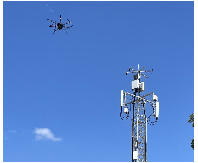
Fig. 4: The UAV during flight and fixed node (tower).
