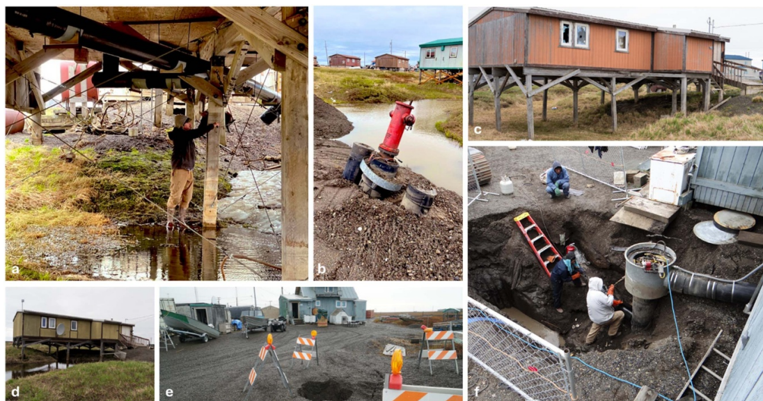
Figure 2. Interactions between degrading permafrost and infrastructure in Point Lay (Kali), Alaska. (a) Where residential pilings were founded in ice wedges, nearly 2 m of thaw subsidence has occurred below some homes leaving less than 1 m of pile embedment (Photo: Peppi Bolz). (b) Thermokarst has disconnected several of the fire hydrants in the northern portion of the community (photo: Benjamin Jones). (c) A North Slope Borough Housing Authority home that has been abandoned due to ice wedge thermokarst (Photo: Billy Connor). (d) A residential home in Point Lay (Kali) showing differential thaw settlement (Photo: Billy Connor). (e) A sinkhole on a residential street associated with underground thermal erosion due to a waterline failure (Photo: Bill Tracey Sr.). (f) Water and sewer utility failure at a home in Point Lay (Kali) (note the exposed ice wedge to the left of the maintenance crew) (Photo: Bill Tracey, Sr.).
