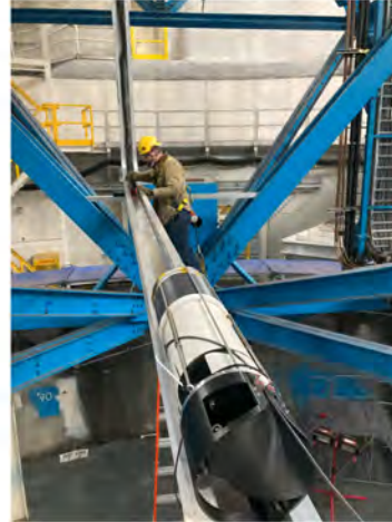
Figure 9. Left: Fiber path (in green) from the Keck I AO room (FIU location) to the observatory basement (spectrometer location). The telescope azimuth cable wrap is indicated, but was avoided through the use of a significantly smaller KPF-specific fiber wrap. Center: Installing the KPF fibers within the fiber trays mounted on the telescope. Within the vertical section a Triflex carrier can be seen; after the fiber cables were installed within it, the Triflex was twisted into a slow helix. This increased the internal friction in the fiber cables by adding a continuous weak bend, and was employed for the vertical sections of the route to prevent the optical fibers from sliding downwards within their protective tubing. In the foreground sits a spool of fiber cable waiting to be installed; these spools had to be custom-designed to pass the coiled-up fibers through the smallest aperture along the route. Right: The top end of the torsional fiber cable wrap which connects the rotating telescope to the fixed floor of the observatory.
