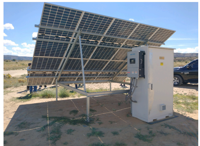
Fig. 1. Image of the type of off-grid solar system considered in this work. The 8 kW inverter, charge controllers, 48 V battery bank and data acquisition system are in the enclosure in the foreground. The bi-facial 3.8 kW PV array tilted at 35 degrees in the background (Louie et al., 2023).
