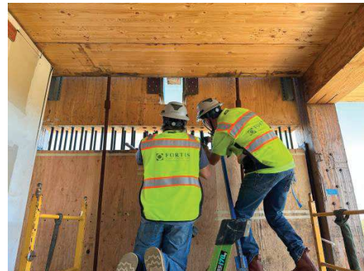
Figure 3. MPP shear wall mating: top panel slowly lowered down as loose rods are aligned.
