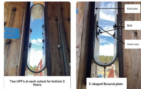
Figure 4: U-shaped Flexural Plate Detail
