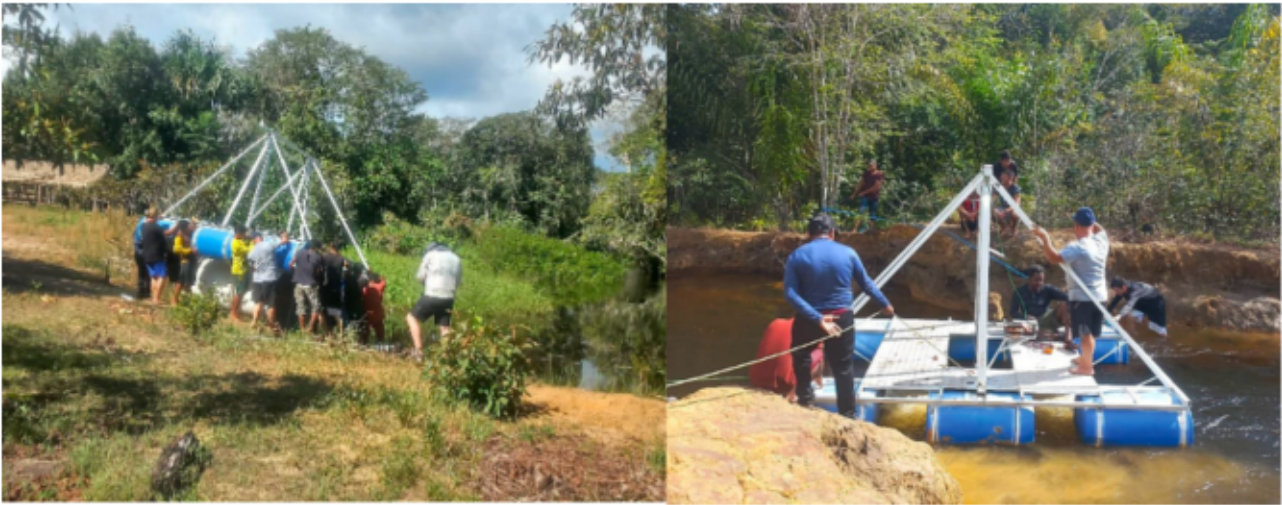
Fig. 6. Process of co-implementation of the in-stream turbine at the community of Cachoeirinha do Mentaí. Researchers and community members worked together to assemble, test and install the turbine (Photos: Karina Ninni).
