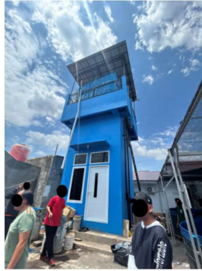
Figure 3. Installed water tower and tank.
