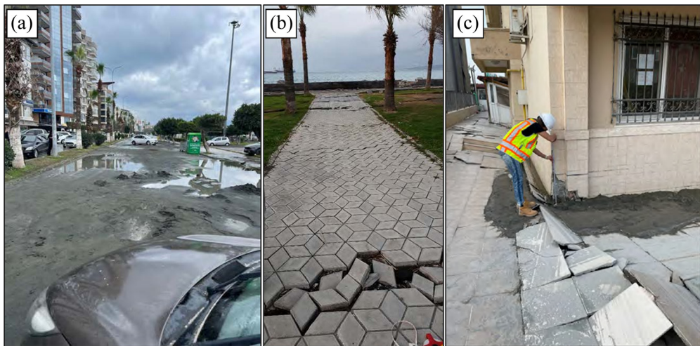
Figure 7. Examples of (a) ejecta along Atatürk Boulevard (delineated in Figure 6) after the M_w 7.8 earthquake, (b) lateral spreading toward seawall at LS4 site, and (c) liquefaction-induced building settlement near Area 1 (from Cetin et al., 2023).
