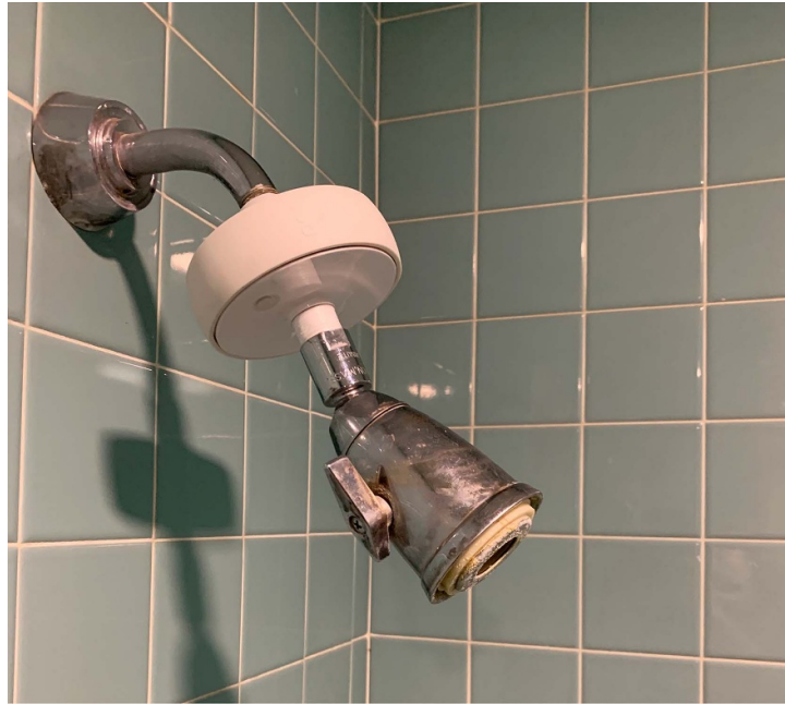
Figure 1. Pani Smart Water Monitor installed on a university shower fixture. (Photo credit: authors).
