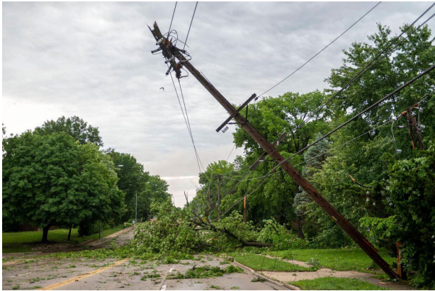
FIGURE 1. Damage from natural disasters, such as damage caused by a tornado as shown here [8], can cause short-circuit fault events.
